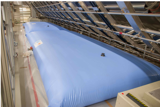
Fig. 8 Two of the four flexible water tanks placed beneath the MS during the gamma suppression measurements.
