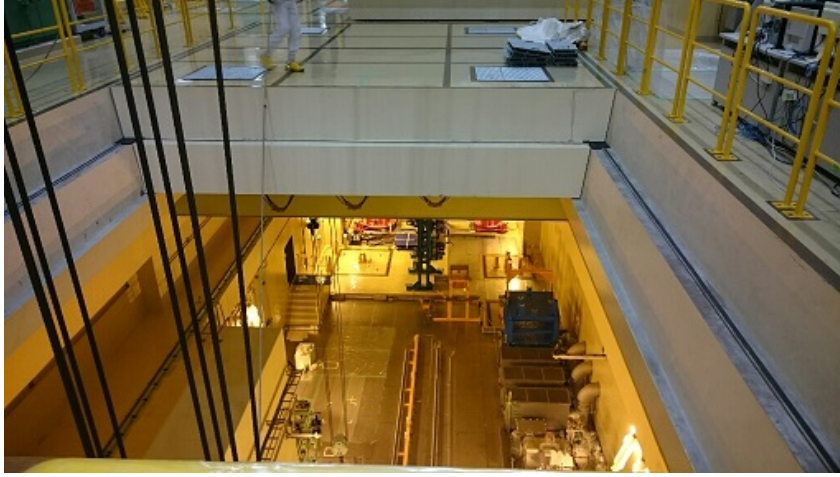
Figure 25: The gum lines are located under the hatches.
