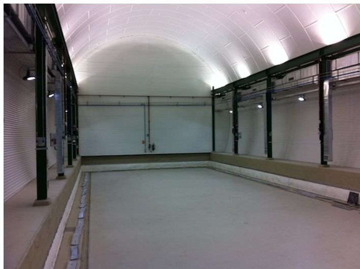
Figure 17. View of Hall A of the Laboratorio Subterráneo de Canfranc prior to any equipment installation.
