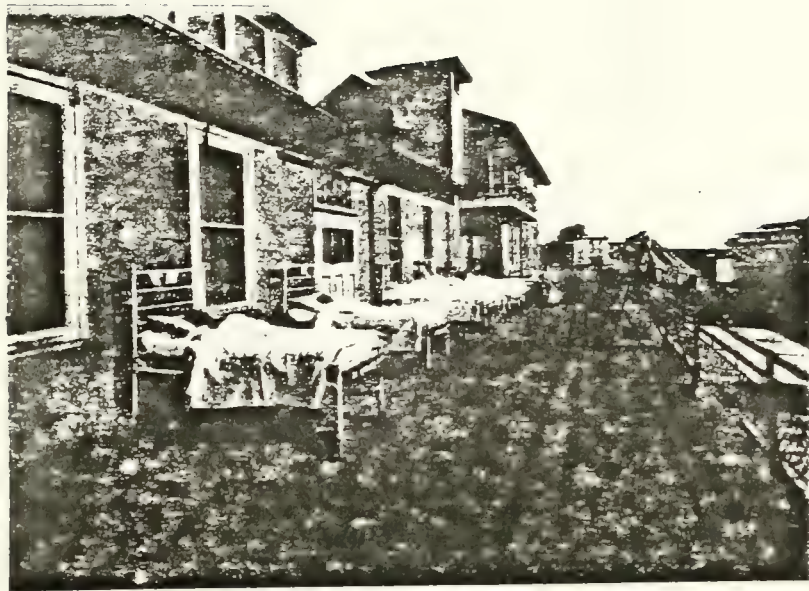
FIG. 21. AIRING BALCONY, PAVILION "C," PETER BENT BRIGHAM HOSPITAL BOSTON, MASS. Codman & Despradelle, Architects.
