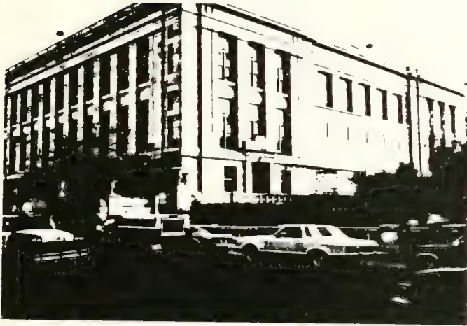
BUILDING "D" FROM LONGWOOD AVE.
