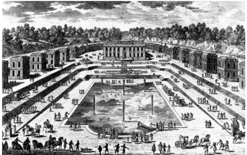
Fig. 70 Adam Perelle. Garden view of the Château de Marly, 1683/84
