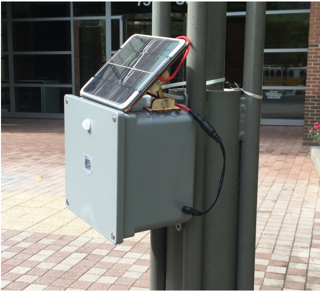
Figure 3. The final LAMBS prototype enclosure mounted on a lamp post.
