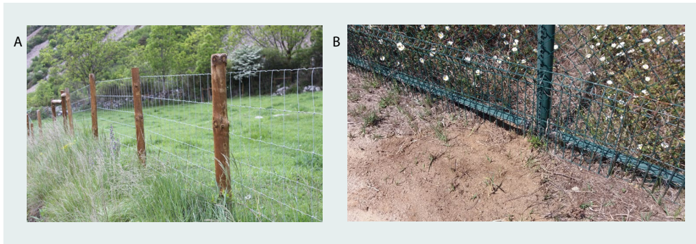
Figure 8.3. Some examples of wild boar proof fences: (A) knotted fences suitable for mitigating damage to pastures are deployed in Catalonia, Spain (photo: C. Rosell); (B) reinforcement fence installed on an existing perimeter fence (photo: F. Navàs).
