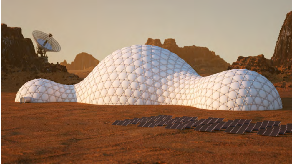
Figure 8: Inflatable freeform dome for a potential Mars habitat.
