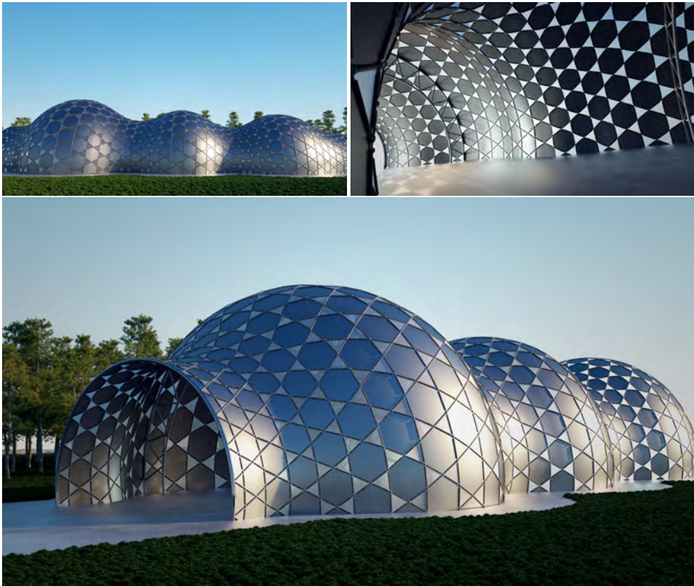
Figure 9: A hybrid shell structure integrates planar support arches in the interior into a deployable auxetic surface.
