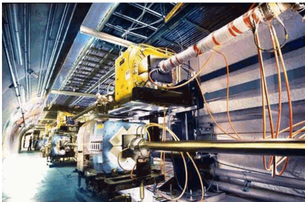
Figure 1 View of the PEP-II tunnel.
