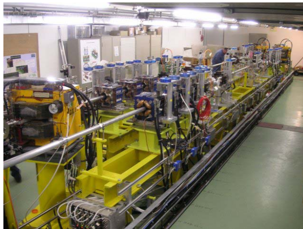
Figure 3: Photo of the TBTS installation.
