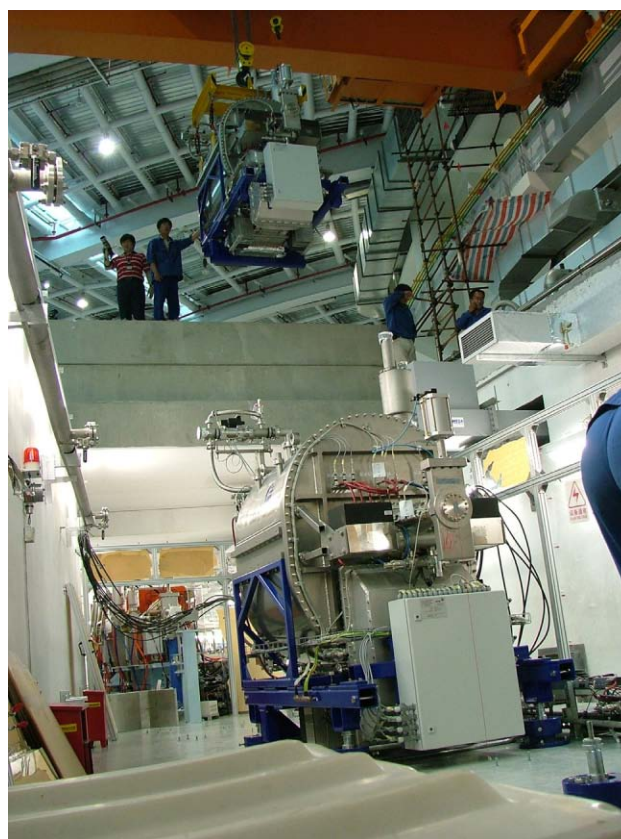
Figure 6: Installation of 500 MHz SRF modules into the storage ring at Shanghai Light Source.
