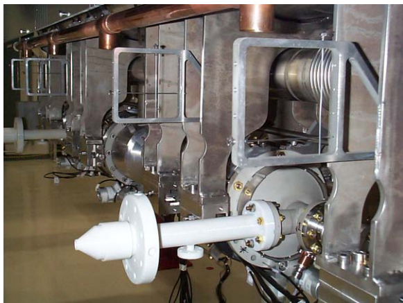
Figure 3: Special alignment panels (found on both sides).
