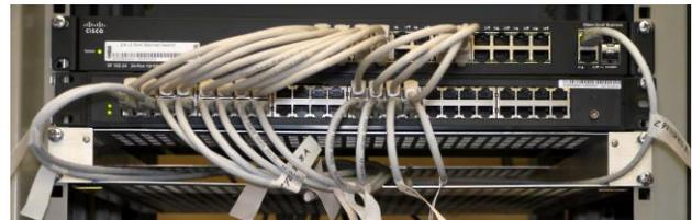
Figure 2: FGC\_Ether star-point with switch and EPI.
