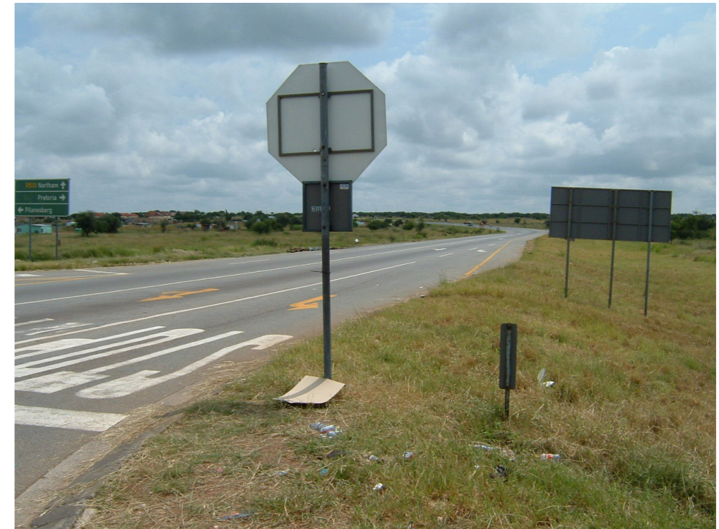
Fig.2.24 Existing Road (R510)
