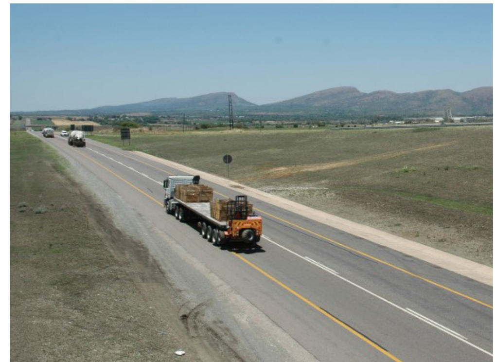
Fig.2.25 Existing Road (N4)
