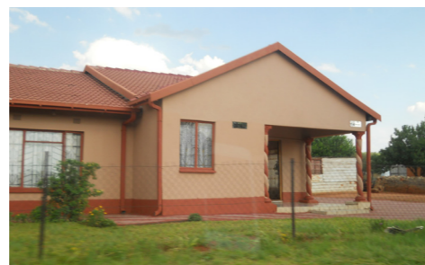
Formal Concrete Blocks
