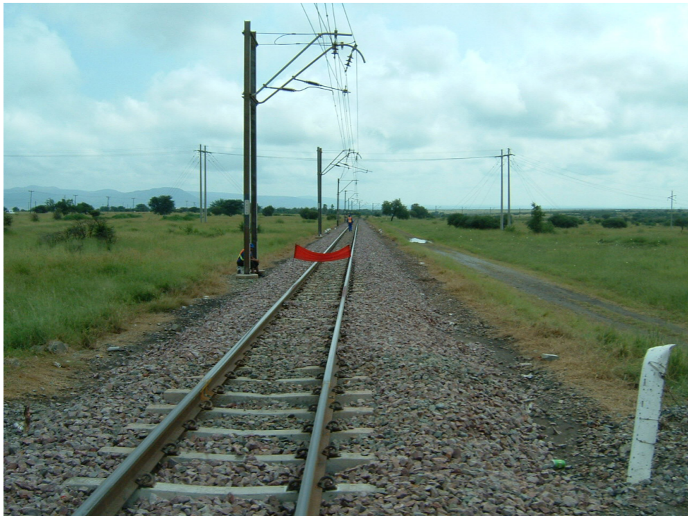
Fig.2.26 Existing Rustenburg Railway
