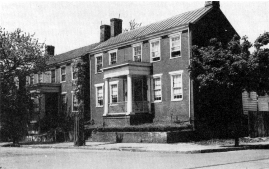
RICHARDSON HOUSES Built 1843 and 1847
