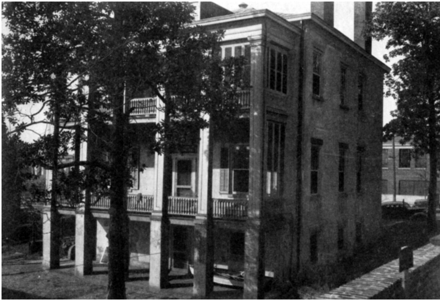
REAR PORTICO OF THE BARRET HOUSE
