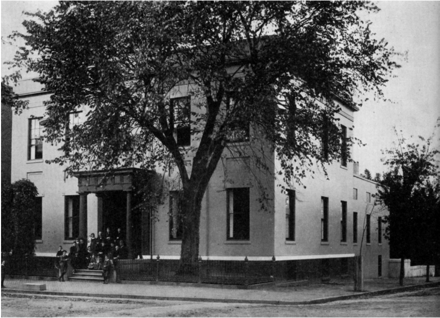
JAQUELIN HARVIE HOUSE Built 1817—Demolished 1906
