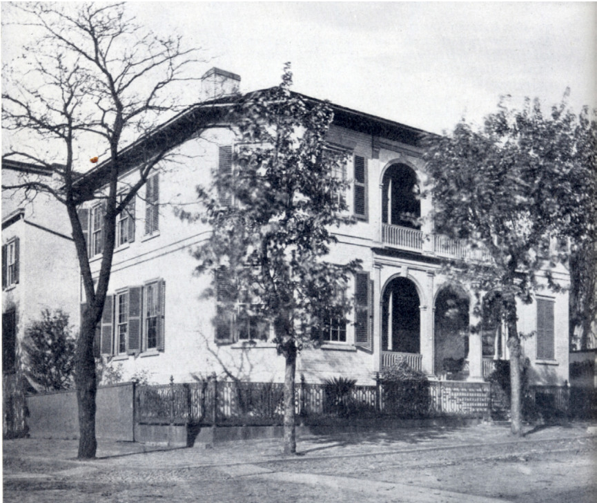
Michael Hancock House Built 1808-09
