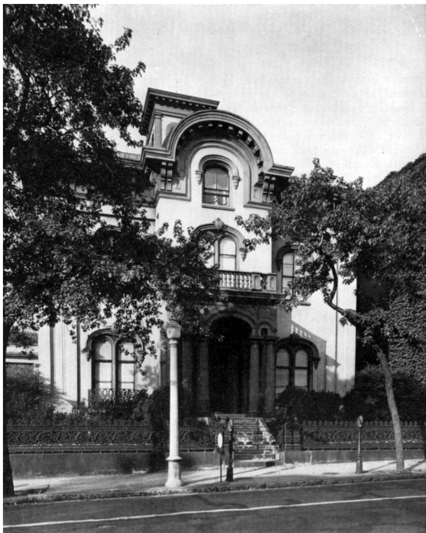
BOLLING HAXALL HOUSE Built 1858
