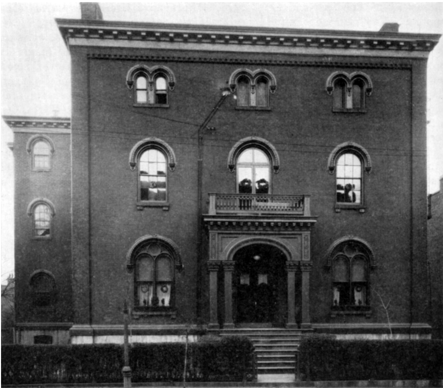
WILLIAM H. GRANT HOUSE Built 1857
