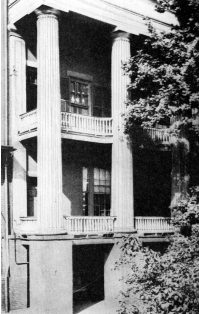
REAR PORTICO, HOBSON-NOLTING HOUSE
