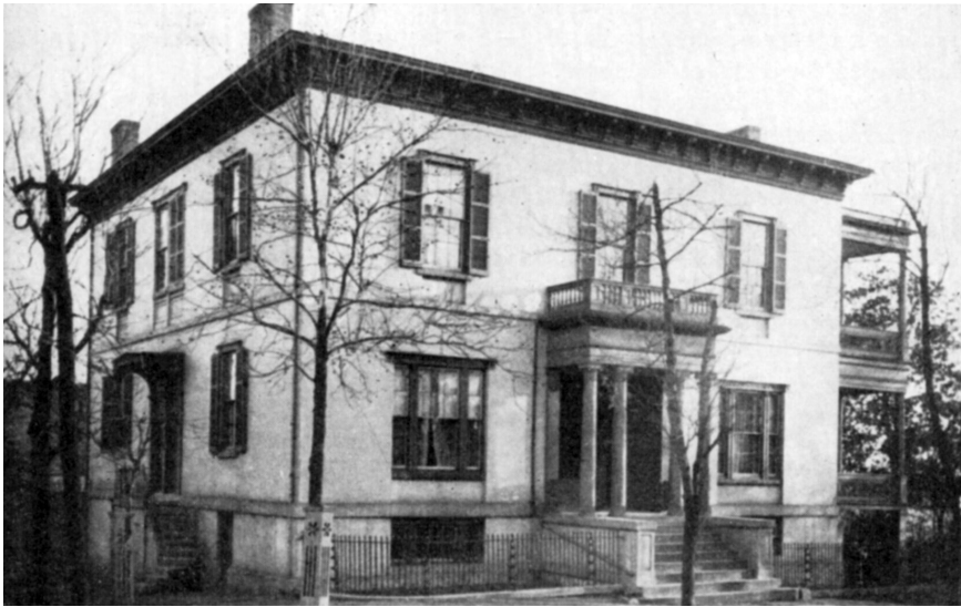
MARX-FREELAND HOUSE Built 1813-14—Demolished 1891
