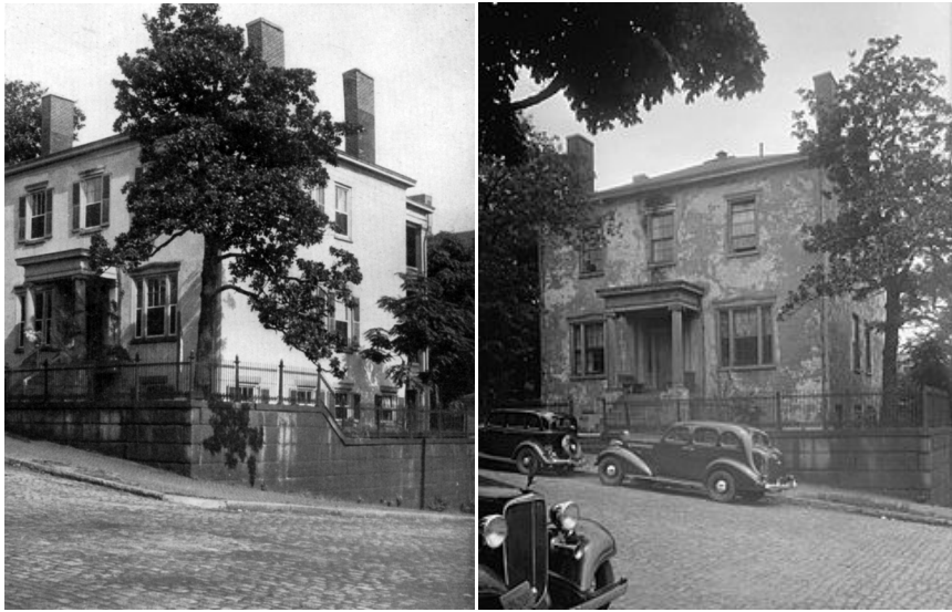
BARRET HOUSE Built 1844
