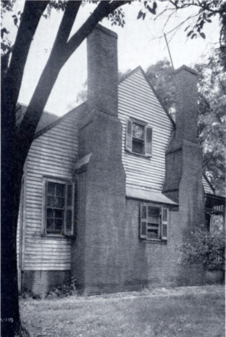
CHIMNEYS OF THE BOTT HOUSE
