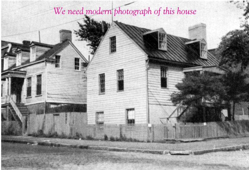
JOHN MORRIS COTTAGES Built 1830 and 1835
