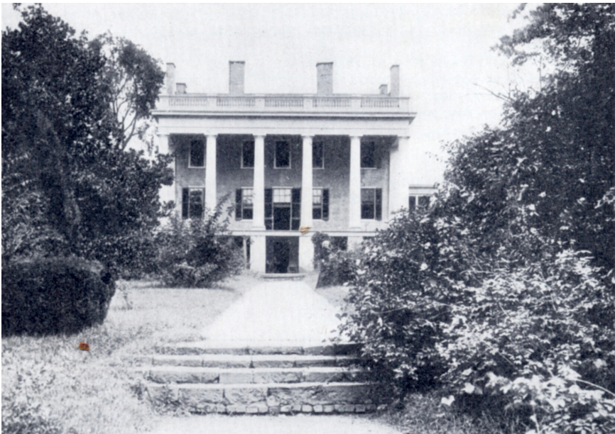
ADAMS-VAN LEW HOUSE Garden side, overlooking the river
