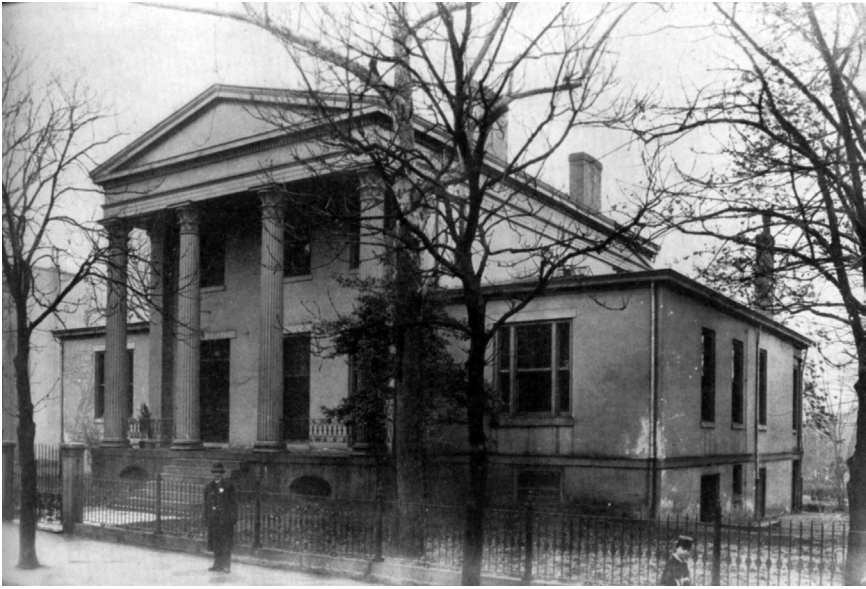
JOSEPH R. ANDERSON HOUSE Built 1845—Demolished 1893
