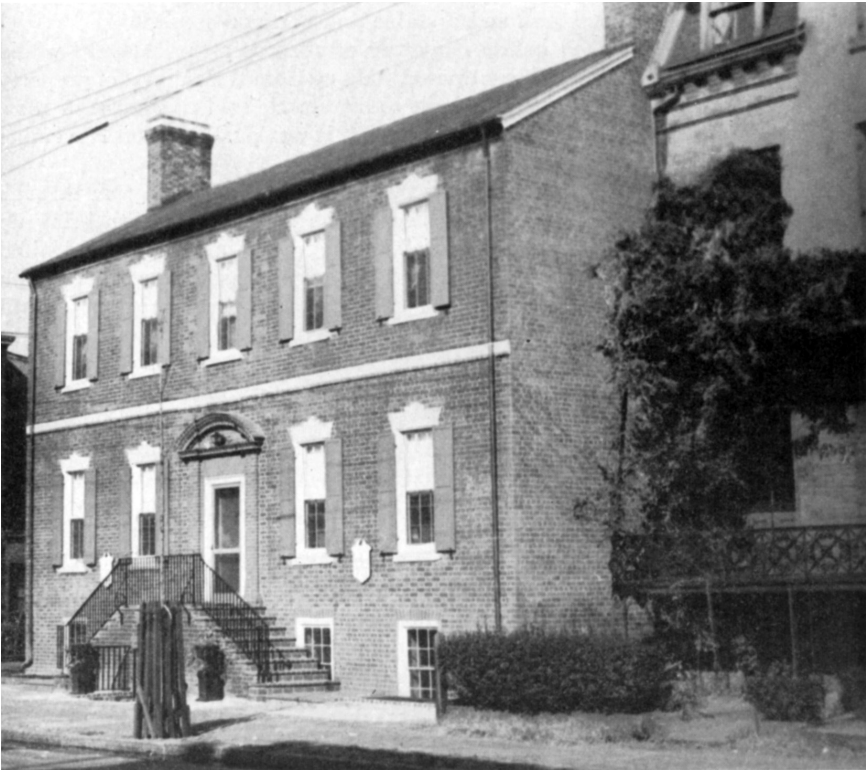
CURTIS CARTER HOUSE After Restoration—Built 1814
