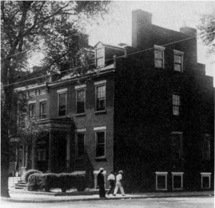
21 WEST CLAY STREET
