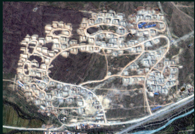
New Jiama (Gyama) Valley Resettlement Village. A total of 144 planned housing compounds were identified from imagery recorded on 8 August 2012. Approximately 73% of building foundations were under construction at this time. 29° 46' 0.495" N 91° 40' 10.991" E © 2013 DigitalGlobe. Source: e-geos
