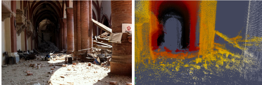
Figure 3.6: Comparison of the point cloud reconstruction with a photograph taken during exploration. Left: Photograph of the western gallery with the collapse roof on the right. Right: Front view of the reconstruction.
