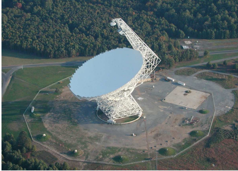
Figure 2: Photograph of the 100 m Robert C. Byrd Green Bank Telescope (GBT) located at the National Radio Astronomy Observatory (NRAO) site in Green Bank, West Virginia. The GBT is the largest fully-steerable single-dish radio telescope built to date, and has a collecting aperture of 110 \times 100 m.
