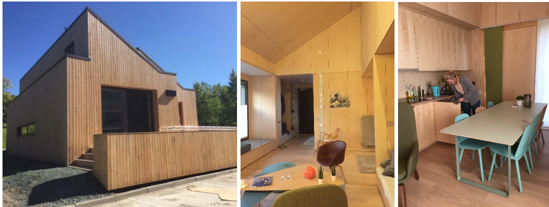
Figure 1: Exterior and interior images of Living Lab, photo SINTEF Building and Infrastructure, 2015
