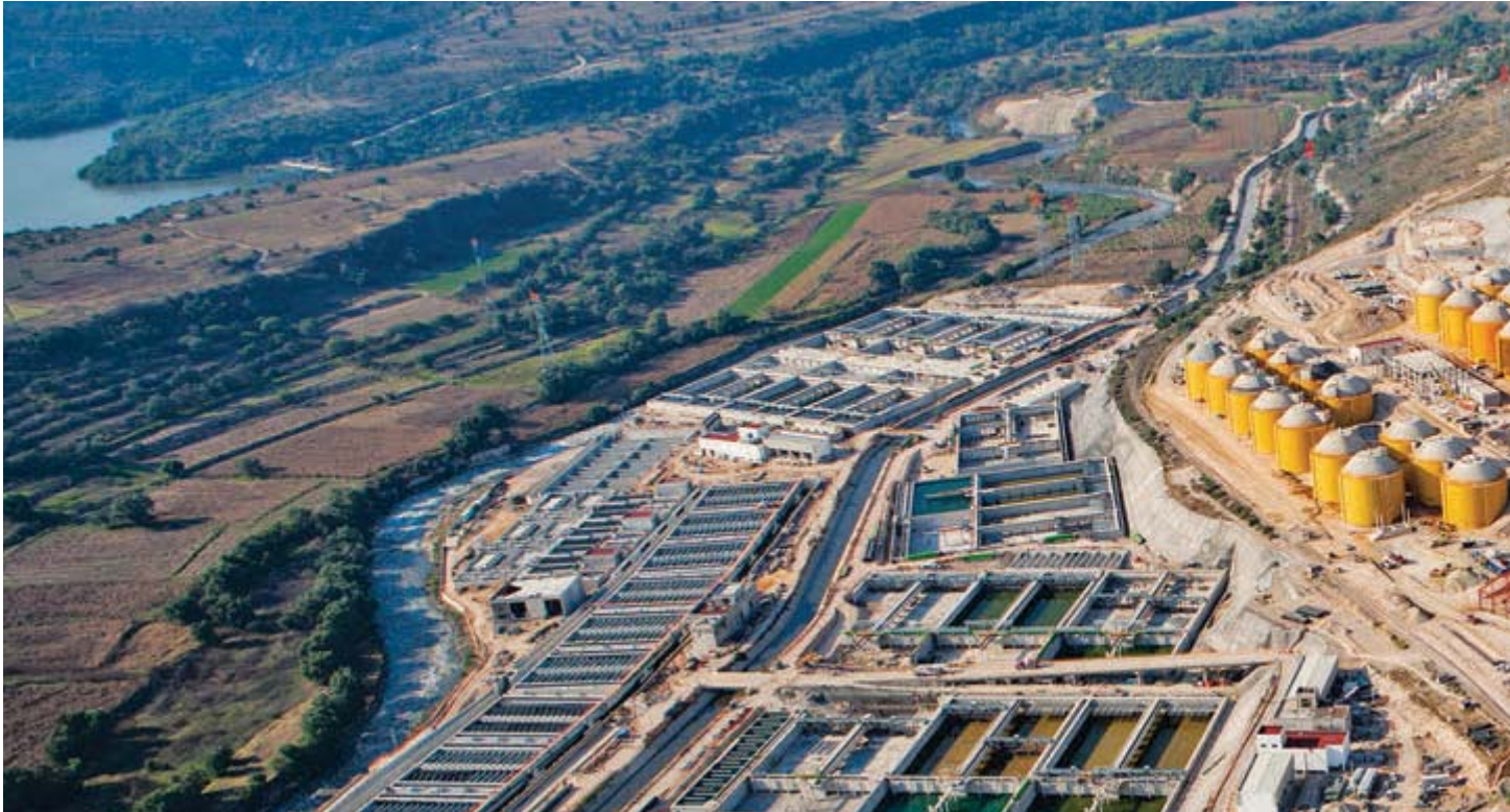
Atotonilco Wastewater Treatment Plant (the largest of its type in the world), Hidalgo.
