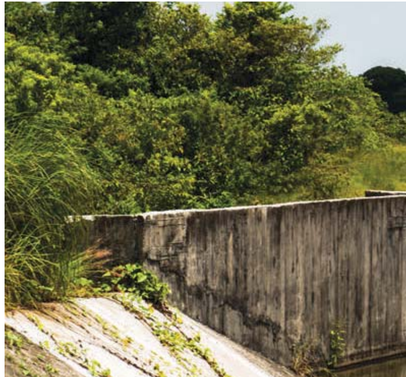
Conveyance channel, La Cangrajera Dam, Veracruz.
