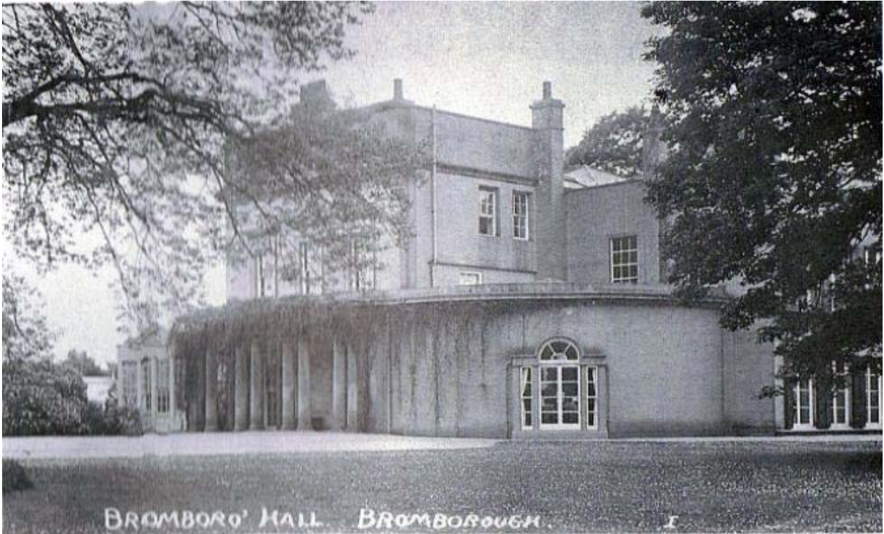
Bromborough Hall Front View
