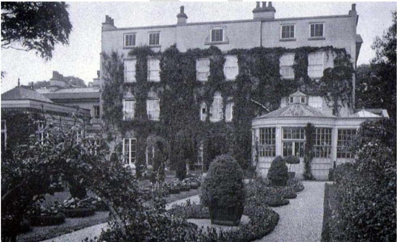
Bromborough Hall Rear View
