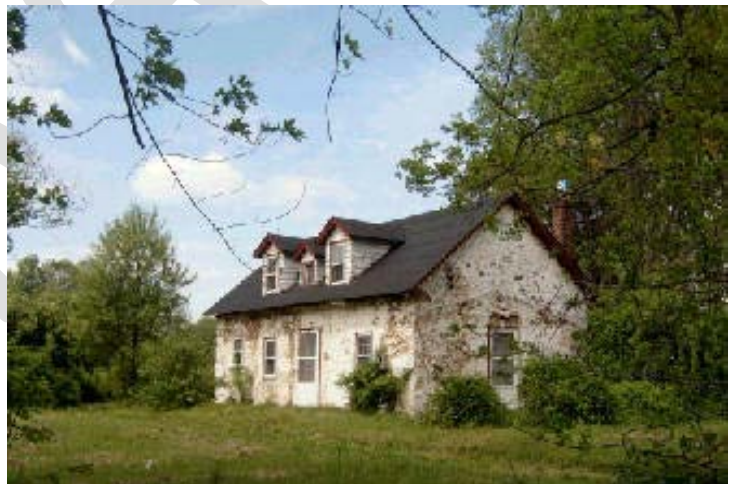
The building off Silerside Road as it appears today in 2003, one of the nation's first free public schools.
