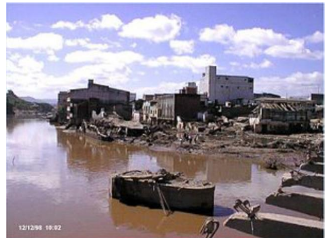
Part of the massive damage caused by Hurricane Mitch in Tegucigalpa, 1998.
