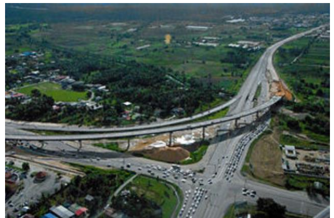
An intersection of Churchill–Roosevelt Highway and Uriah Butler Highway, 2009
