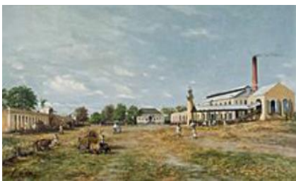
Hacienda La Fortuna . A sugar mill complex in Puerto Rico painted by Francisco Oller in 1885 (Brooklyn Museum)
