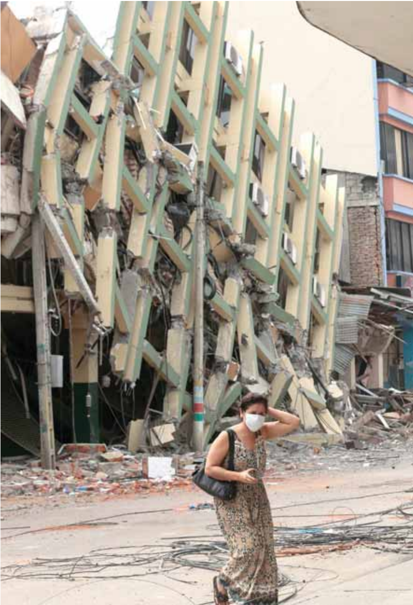
A destroyed building after the April 2016 earthquake hit the town of Portoviejo, Ecuador. PHOTO: AFP
