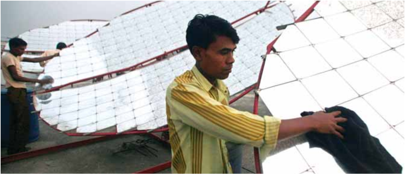
Workers clean solar concentrator panels (solar parabolic dish) at the Tapi solar food processing unit at Kapodra village, India. PHOTO: REUTERS
