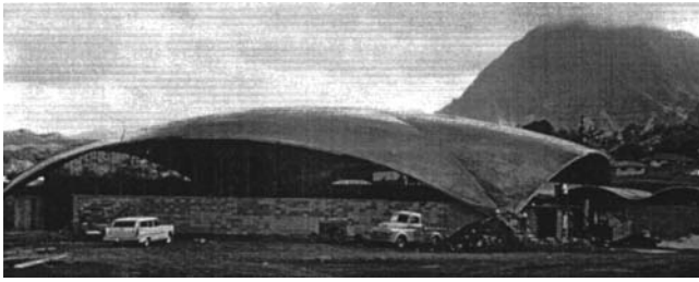
Fig. 13. 64–127 mm (2.5–5 in.) thick, 37 m (120 ft) span intersecting tori with no ribs or hinges (Richard Bradshaw)
