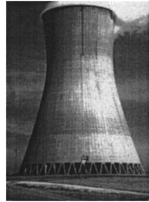
Fig. 15. Cooling tower, generated by straight lines (Gould 1988)
