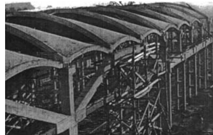
Fig. 16. Conoid, generated by straight line traveling along another straight line at one end and curved line at other end (Joedicke 1963)
