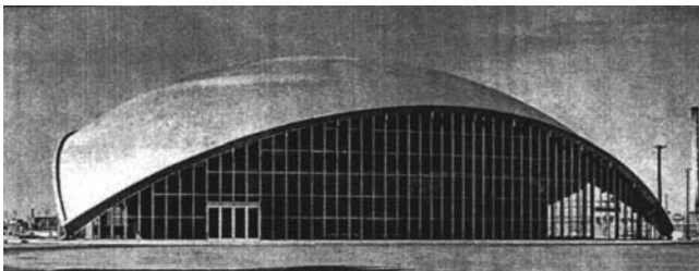
Fig. 7. 89 mm (3.5 in.) thick, 49 m (160 ft) span spherical shell with hinges at abutments, MIT Auditorium, Boston, Amman and Whitney Engineers (Joedicke 1963)
