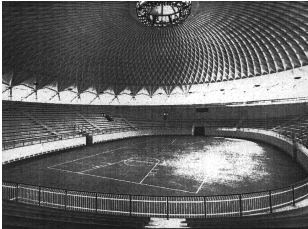
Fig. 10. Inside view of Sports Palace, Rome (coffered ceiling made by pouring a thin layer of concrete over precast concrete boxes which then become part of the structure) (Joedicke 1963)
