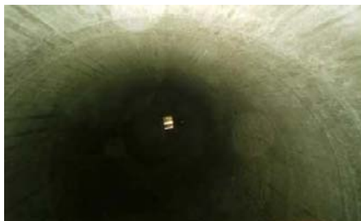
Looking up into Silo #5, one of the silos used in generating the acoustical experience of the Silophone. (Photo by Diana Shearwood. Courtesy of Emmanuel Madden)
