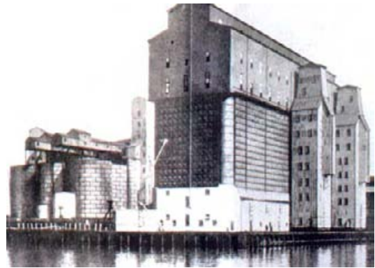
Dakota Elevator with exposed steel bins, praised by LeCorbusier. From W. Gropius, Jarbuch des Deutschen Werkbindes 1913 (Courtesy of the Buffalo and Erie County Public Library)
