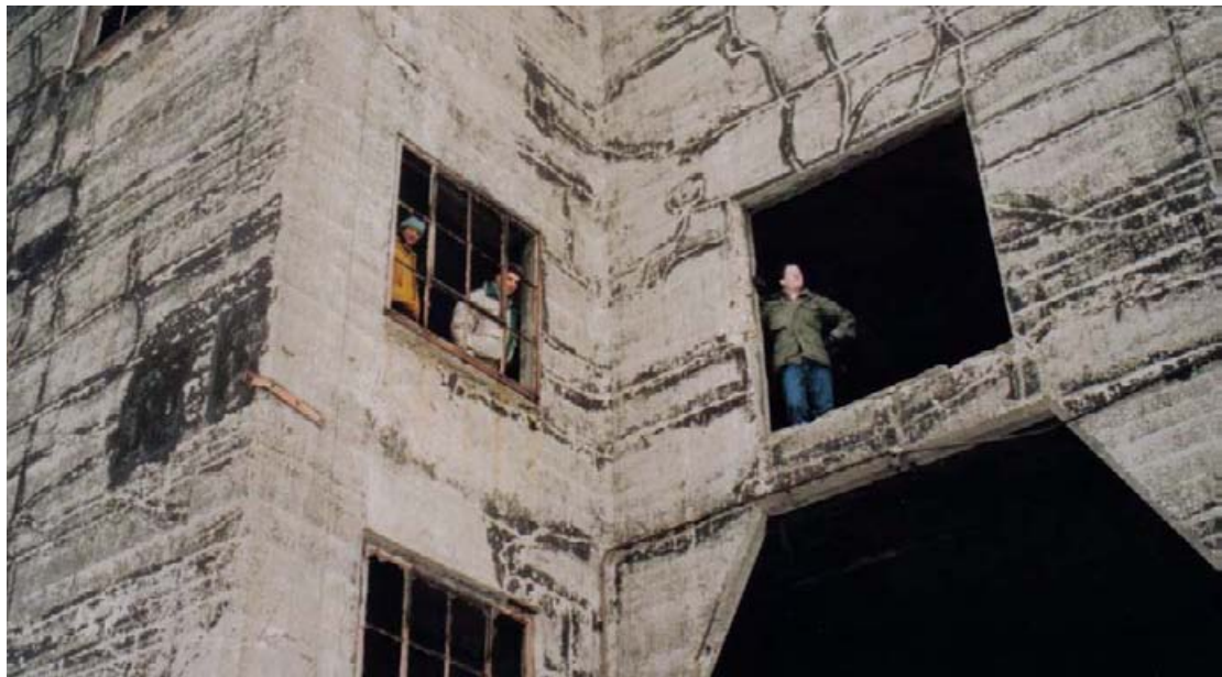
Accessing the elevators is difficult but many find it irresistible. (Photo by Lynda H. Schneekloth)
