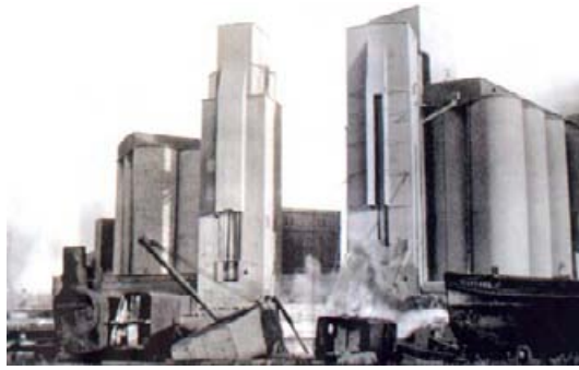
American Elevator (1906), the first concrete elevator erected on the Buffalo River. From E. Mendelsohn, Amerika 1926 (Courtesy of the Buffalo and Erie County Public Library)
