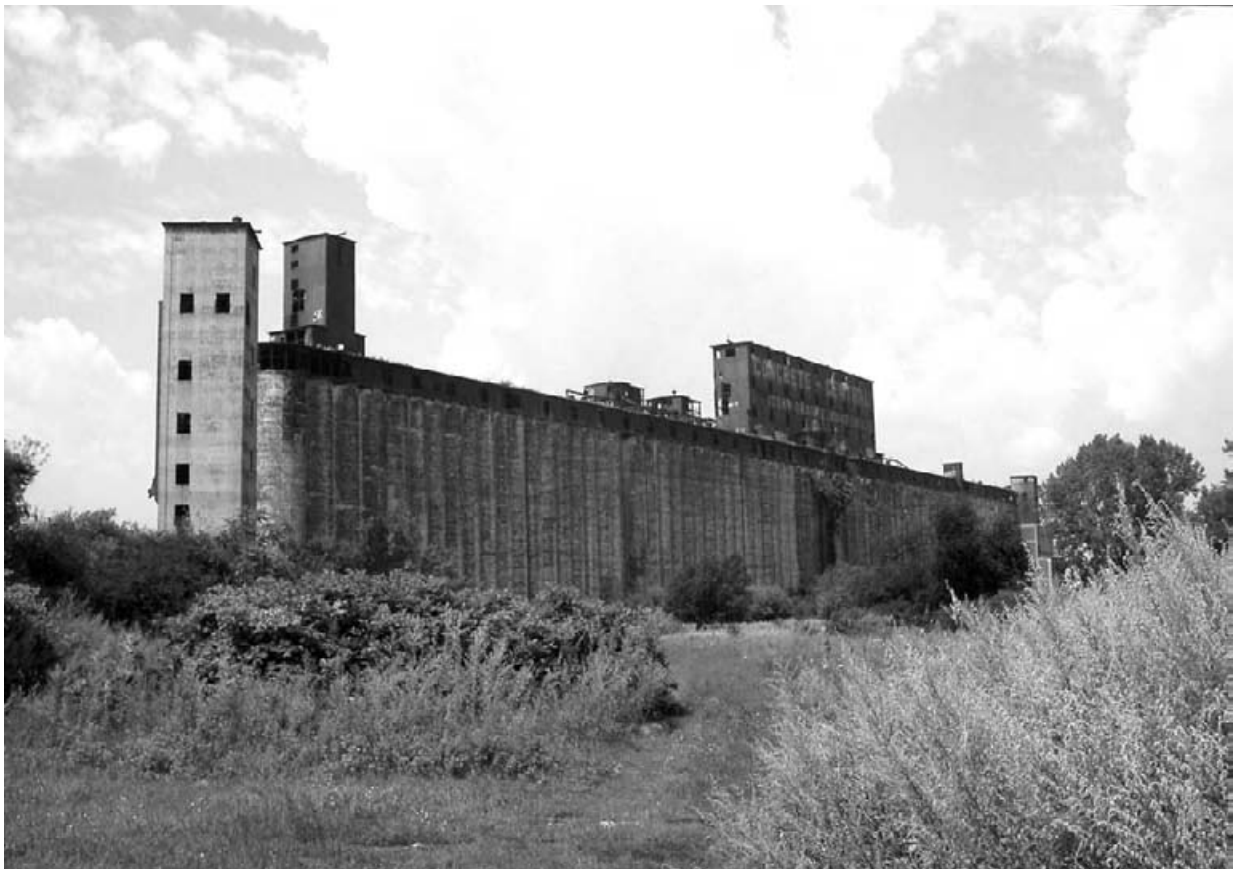
Concrete Central Elevator (Photo by Ivonne Jaeger)
