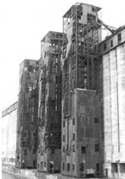
Marine Legs on the Concrete Central Elevator (Photo by Lynda H. Schneekloth)
