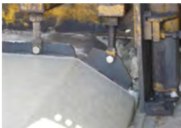
Figure 3.3 Iowa safety edge on PCC
