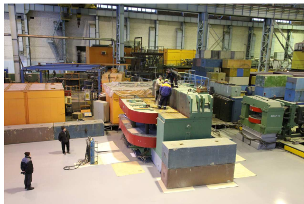
Figure 5.13: The picture of the SP41 magnet dismounting in the 205 experimental hall.
