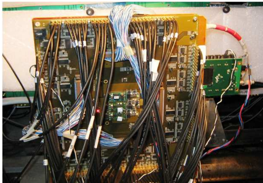
Figure 5.37: Photo of 128-channel TRB (with AddOn board) installed in beam test area to read-out signals from four mRPC prototypes.
