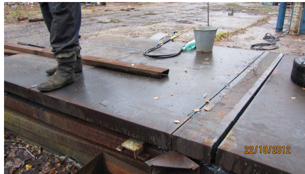
Figure 5.12: The pictures of the steel plates cutting of the SP41 magnet.
