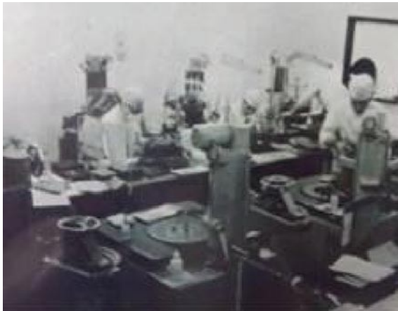
Figure 27 Gauge block lapping (1966)
