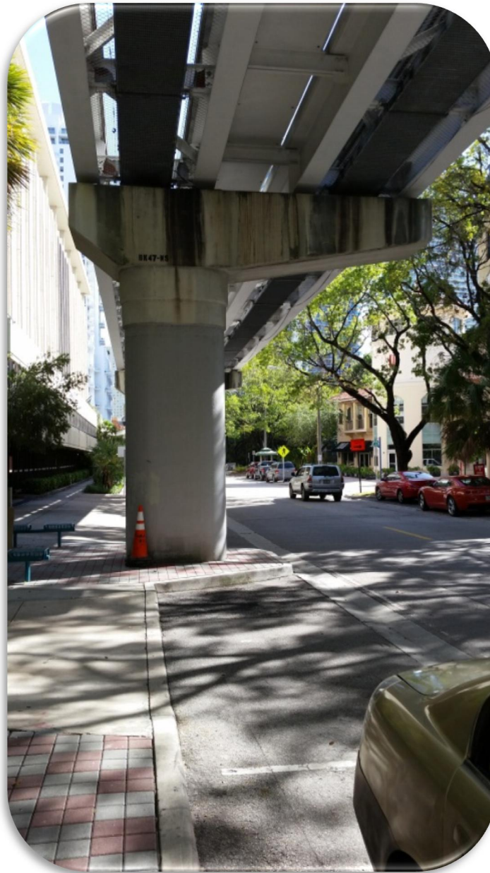
Figure 67: Existing Single Pier Support, SE 1 st Avenue
