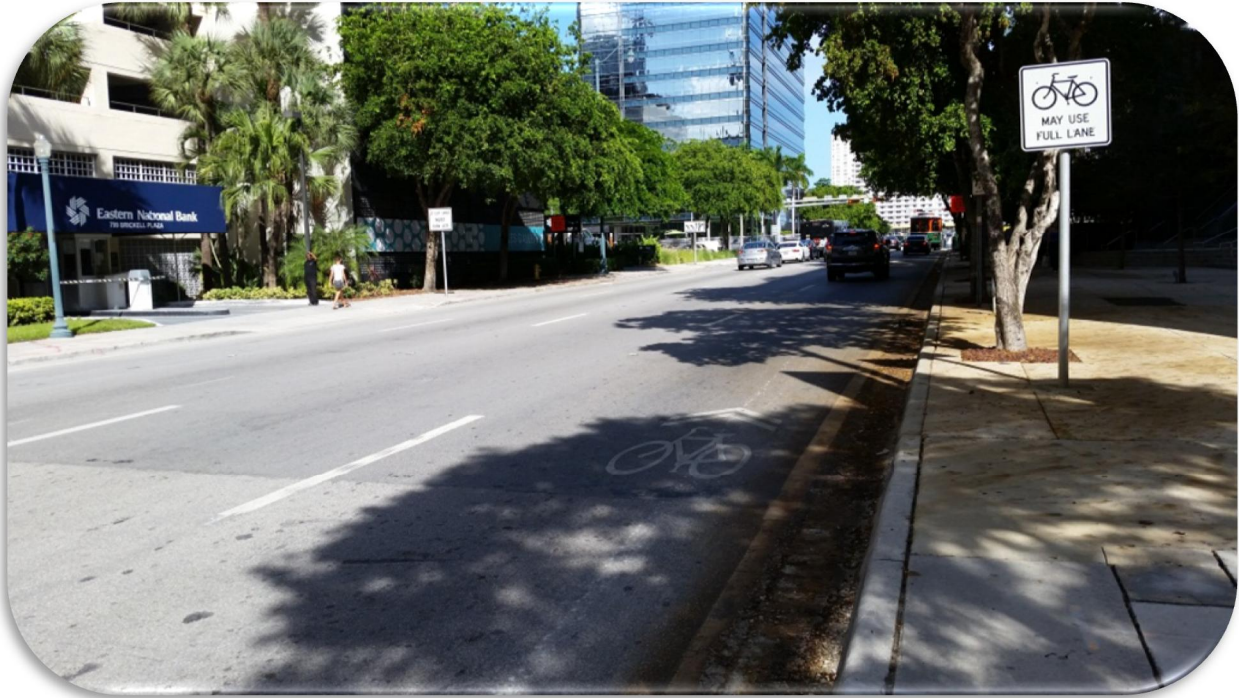
Figure 65: Existing Street View, Cross Section 1
