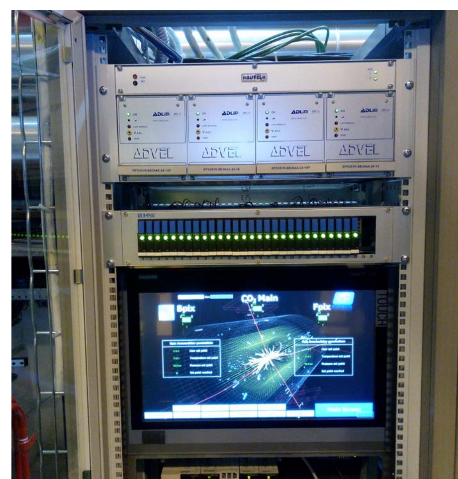
The 24V DC hot-swappable redundant power supply, DC circuit breakers and HMI
