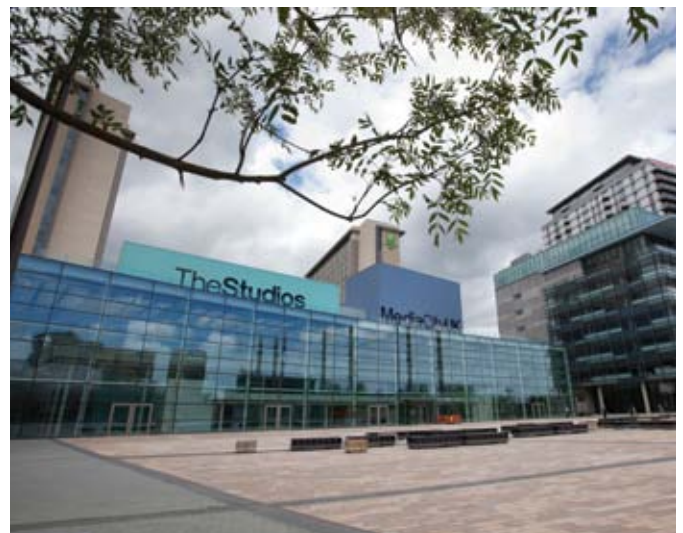
The fit-outs for both MediaCityUK at Salford (shown here) and London's Broadcasting House are delivering on time and under budget.
