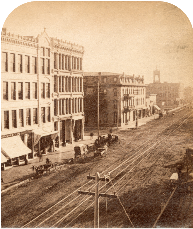
Hennepin Avenue in Minneapolis, as it appeared during the Belmont sensation, 1880.
