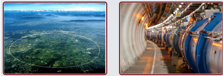
Figure 1: The 27 km LHC tunnel, housing the LHC accelerator, here showing the superconducting magnets containing the two beam pipes. [26].
