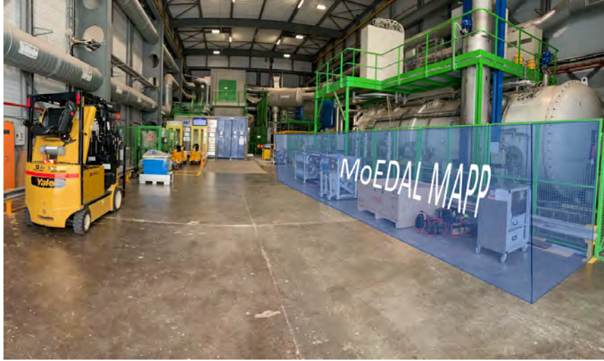
Figure 14: The temporary staging area in SBD 2855.
