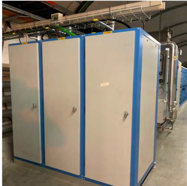
Figure 19: The source of the optical fibres carrying the LHC clock to the MAPP-mCP detector.
