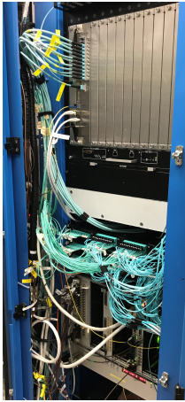
(4a) Fully populated MUCTPI rack in the ATLAS counting room.
