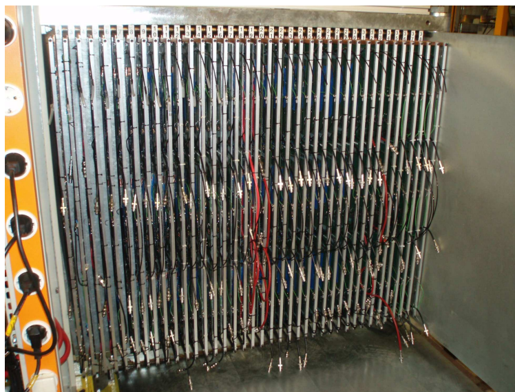
Figure 3. Photograph of the DHCAL stack before cabling.
