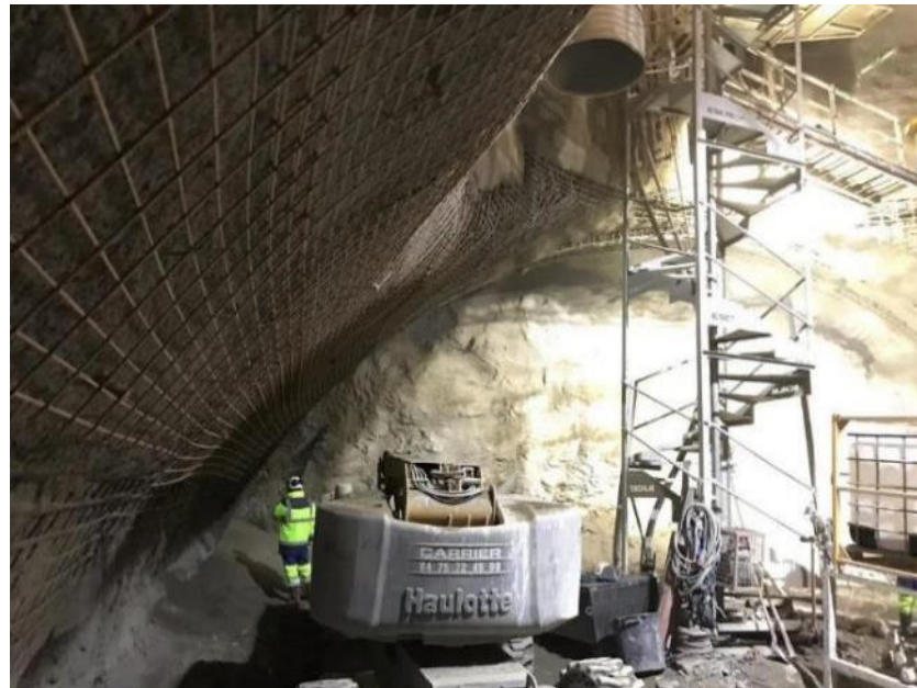
Start of cavern excavation at Point 5
