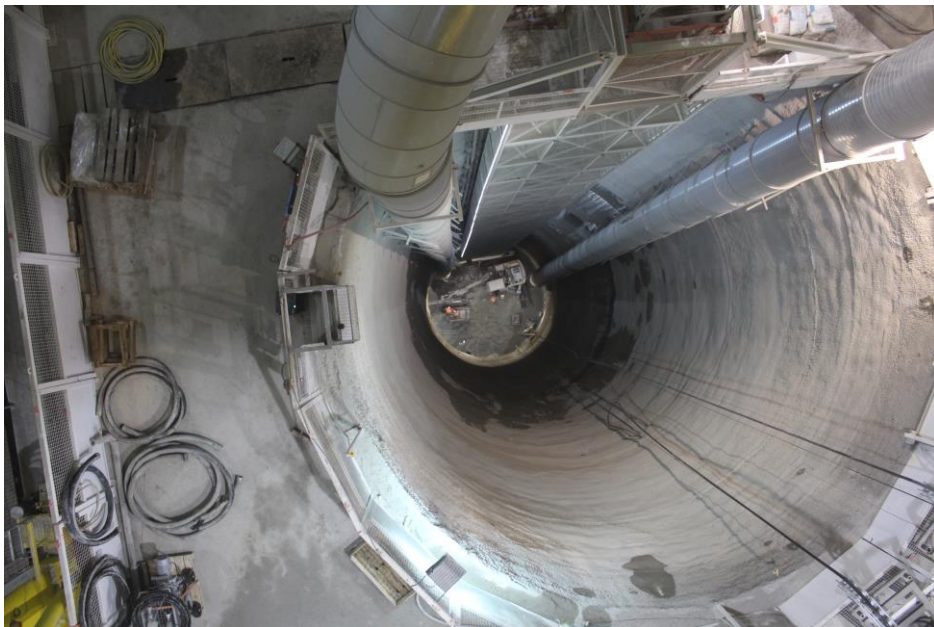
Shaft picture seen from the top
