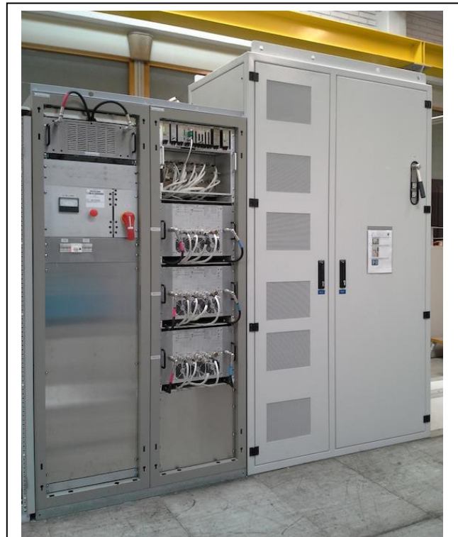
Figure 57: The prototype of the 24 kV power converter, developed by TE/EPC in collaboration with the RF Group, expected to upgrade the performance of the LHC-dedicated 40 and 80 MHz RF systems in the PS.
