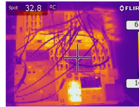
Fig. 6. Thermal picture of the jFEX prototype switched-on on the bench.
