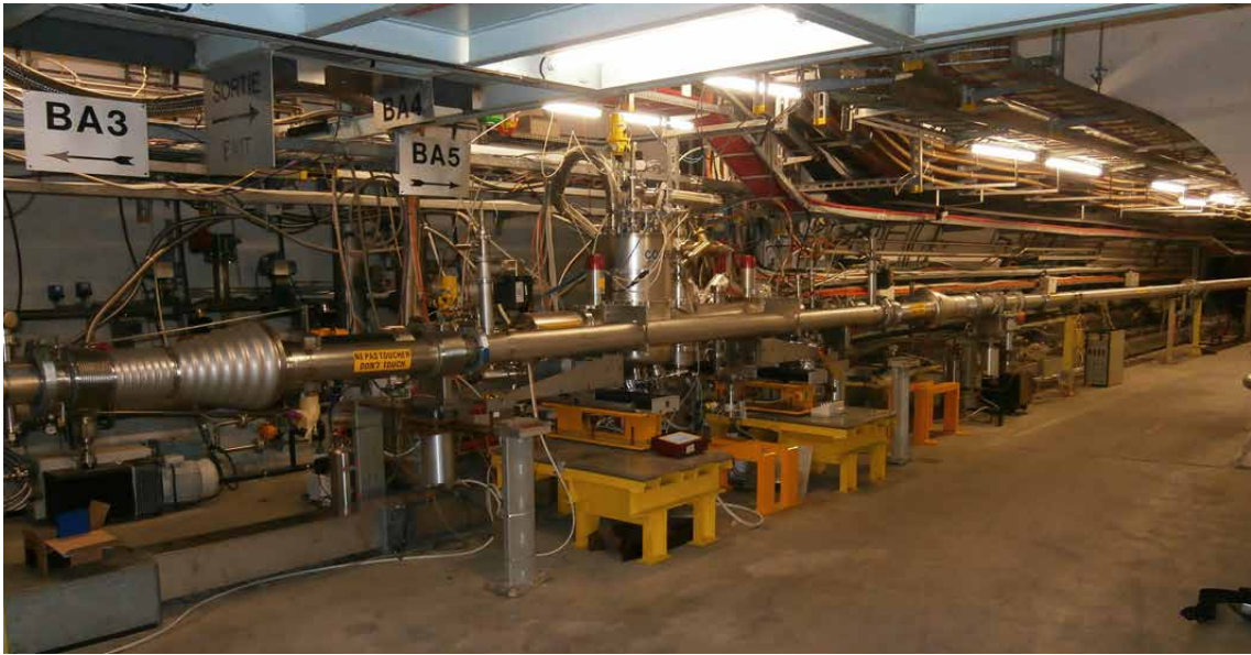
Figure 9.10: Picture of SPS vacuum sectors 430 and 431 installed in TS45 of SPS/LSS4.
