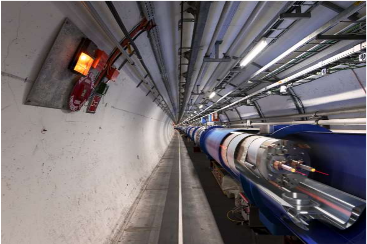
Figure 2: Cross section of the superconducting dipole magnets in the LHC tunnel [2] .
