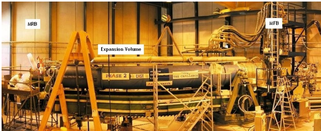
Figure 6-6: Picture of the 'Expansion Volume' being lowered by the crane into its final position on top of the magnet cryostat. At each extremity the expansion volume has conical tapers and for a reduced diameter, passing on the MRB side under the yellow chariot for the vertical movement and of the MFB side under the magnet cooling transfer lines.
