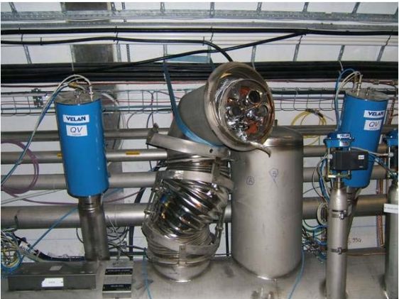
Figure 17: Damage to “jumper” connections of cryogenic distribution line
