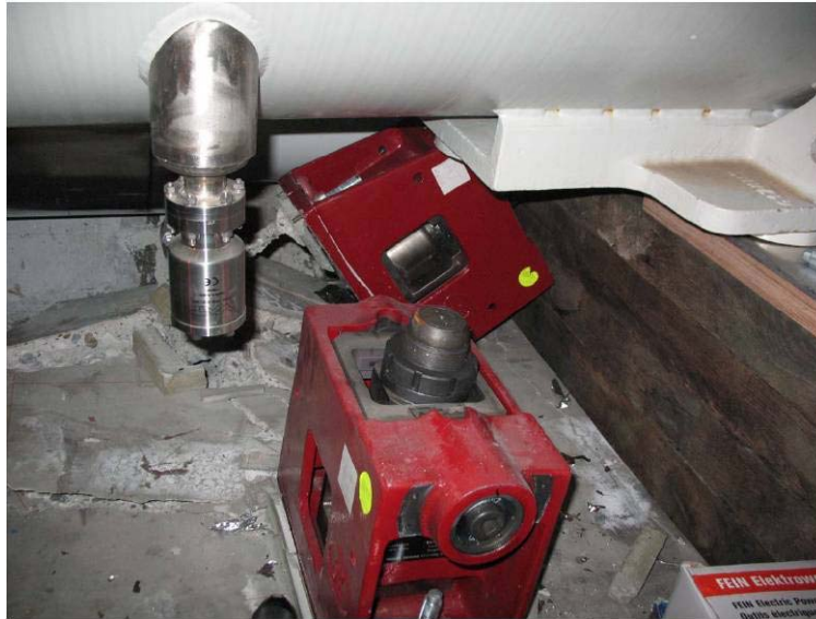
Figure 13: Displacement of supporting jacks and rupture of ground anchors at Q27R3
