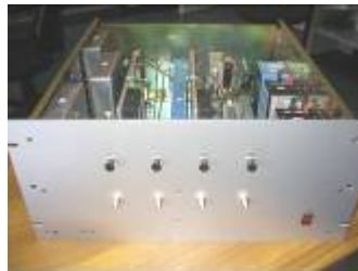
Figure 2: BPM subsystem located in the hall
