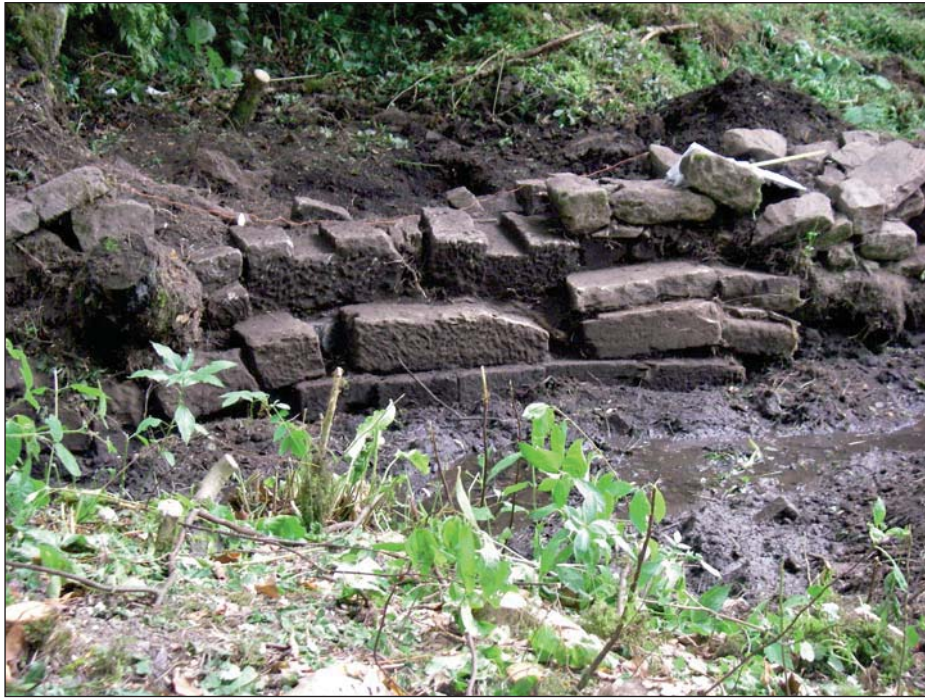
Plate 9: Trench 6, showing wheel-pit wall 6009 with waterwheel fixing points 6003 (view from the north-east; no scale)
