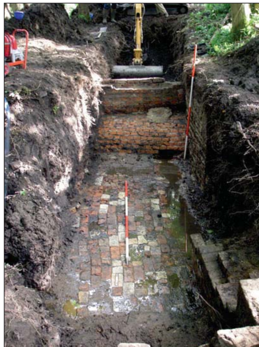
Plate 4: Trench 1 Area B, showing covered tailrace at south end of crucible furnace (view from the south; scales = 2m)
