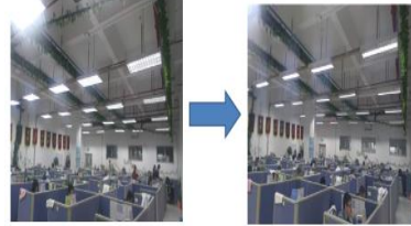
redundant lamp removal
