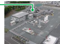
View of pilot plant (within JERA Shin-Nagoya Thermal Power Station)
