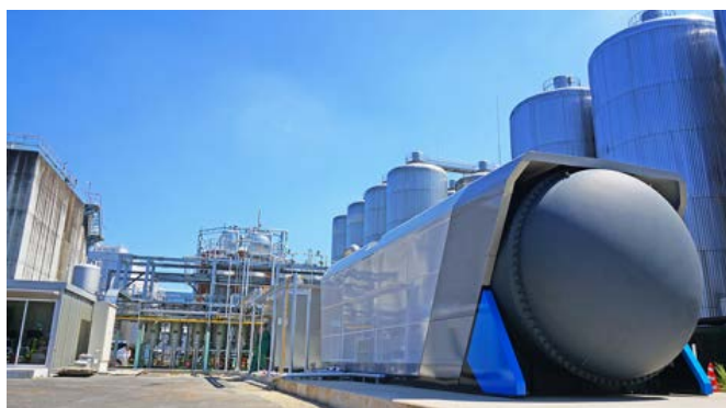
Biogas SOFC at Asahi Breweries Ibaraki Brewery
