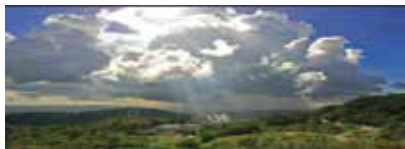
Tongonan Geothermal Power Station
