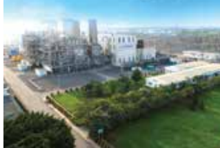
Phu My 1 Combined Cycle Power Plant (1,090MW)
