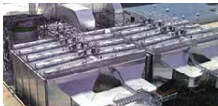
Electrostatic Precipitator for Thai Binh Thermal Power Plant
