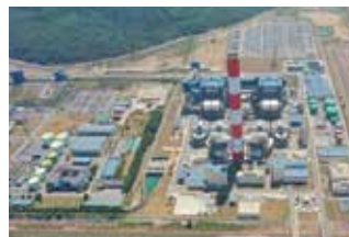
Steam Turbine Generators for Nghi Son 2 Thermal Power Plant (600MWx2)
