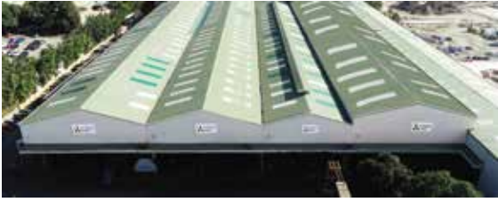
Boiler Factory in Bauan, Batangas
