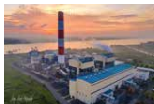
O Mon Thermal Power Plant 1-I (330MW) O Mon Thermal Power Plant 1-II (330MW)
