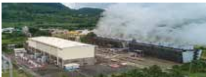
Makban Geothermal Power Station
