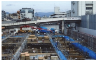
Figure 10 Placement of foundation concrete
