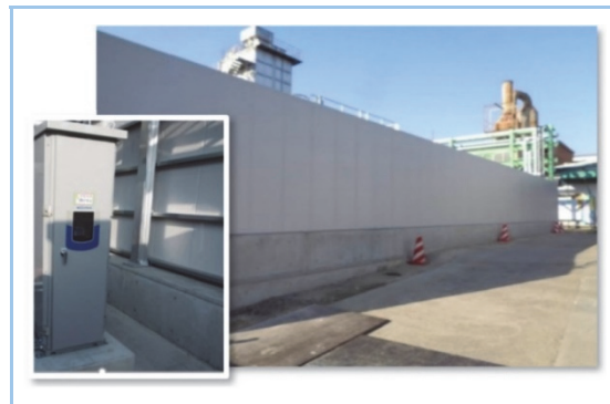
Figure 7 Installation of sound proof walls
