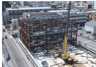
Figure 11 Erection of steel frames
